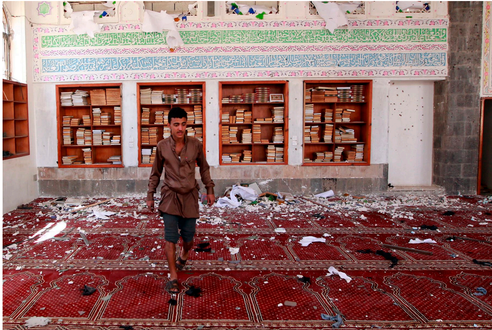
Figure 13.9 A Yemeni man inspects the damage following a bomb explosion at the Badr mosque in southern Sana'a on 20 March 2015 (source: AFP Photo, https://www.ndtv.com/world-news/142-dead-in-yemen-mosque-bombings-claimed-by-islamic-state-748392 )
