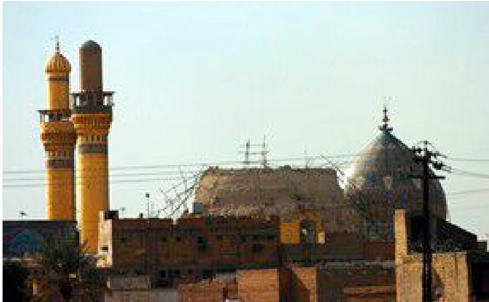
Figure 31.3 The extensive damage to the al-Askari Shrine in Samarra, Iraq in 2006 has been regarded by many as the tipping point that turned general unease with the coalition presence in Iraq into a full scale, sectarian civil war. The minarets were destroyed in 2007. (Photo © US Army, via Wikimedia Commons, https://commons.wikimedia.org/wiki/File:Al-Askari_Mosque_2006.jpg )
