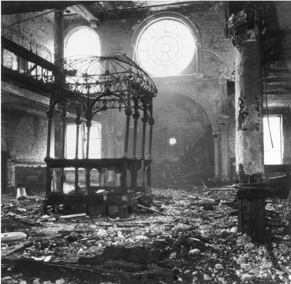
Figure 3.2 The gutted inside of the Nuremberg synagogue after burning and looting by an organized Nazi mob on 9 November 1938
